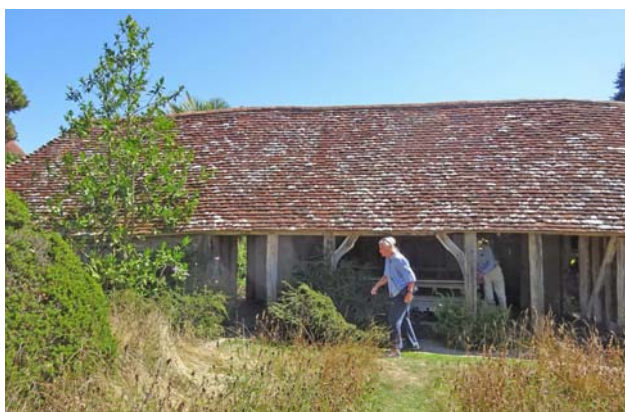
Plate 13 Building 3; opened-up central section of north wall showing inserted posts, braced
