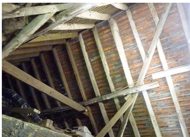
Plate 21 Building 4; Redundant period-A hip at truss A-A looking towards period B extension
