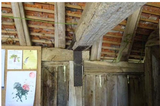
Plate 15 Building 3; stepped joint in wallplate between period A (left) and period B
