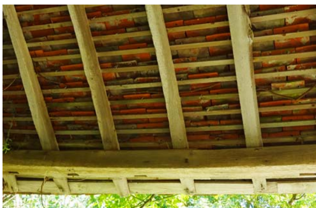
Plate 7 'Loggia'; mortices in underside of tiebeam D-D. Note doorway
