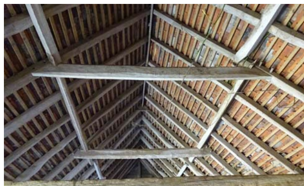
Plate 16 Building 3; roof of central compartment looking east. Note joint between period A and B roofs where the ridgeboard ends
