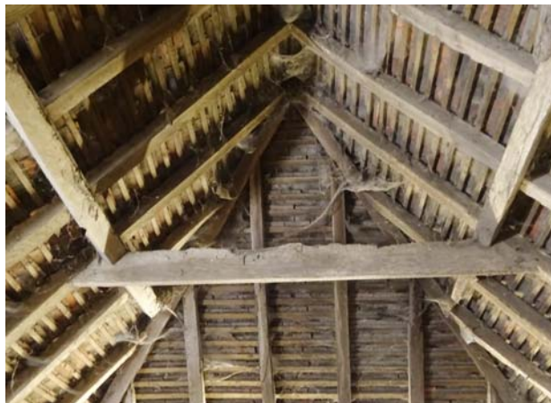
Plate 22 Building 4; Period-A hip looking east showing ends of the clasped side purlins supported by collar
