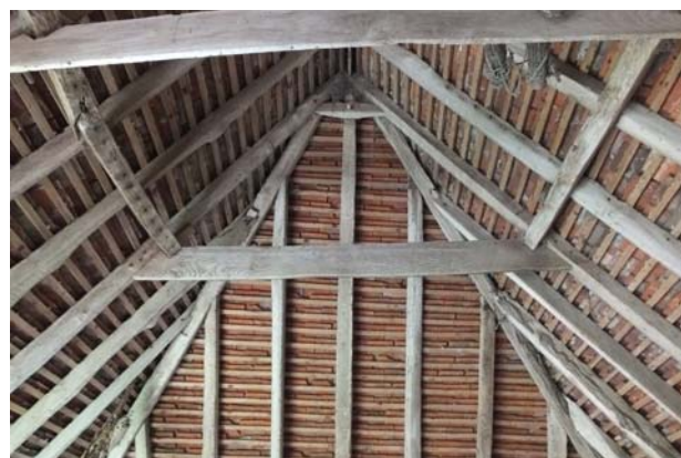
Plate 18 Building 3; reused period-A western hip at western end of period-B extension
