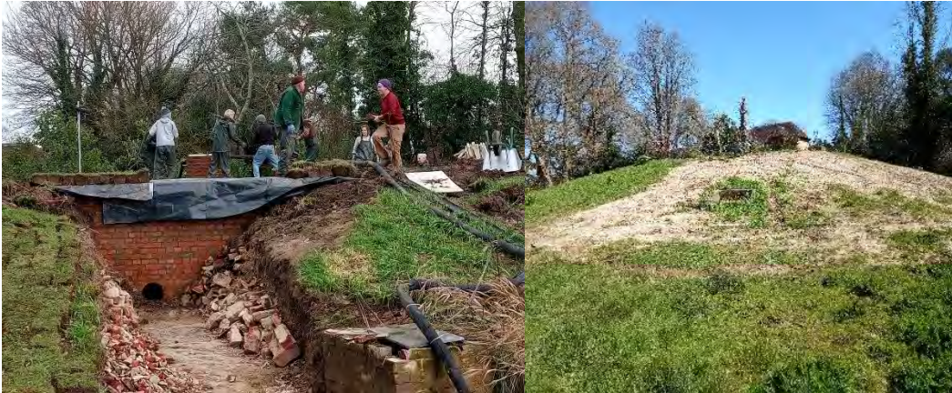
Replacing the turfs on the Reservoir after the repairs
