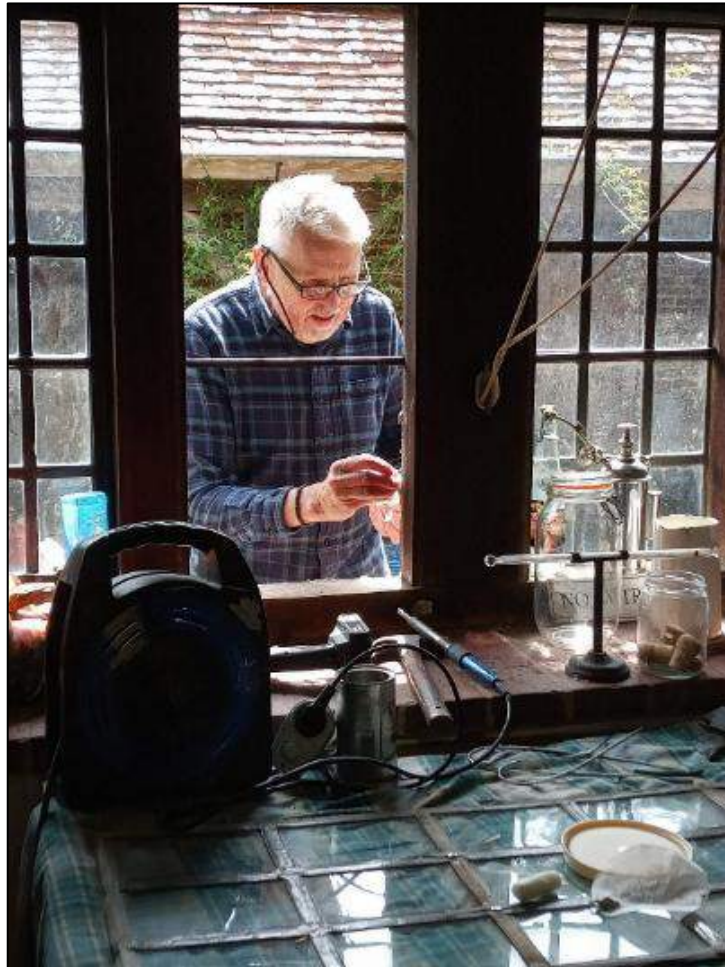
25 Paul Sedgewick repairing the kitchen window.
